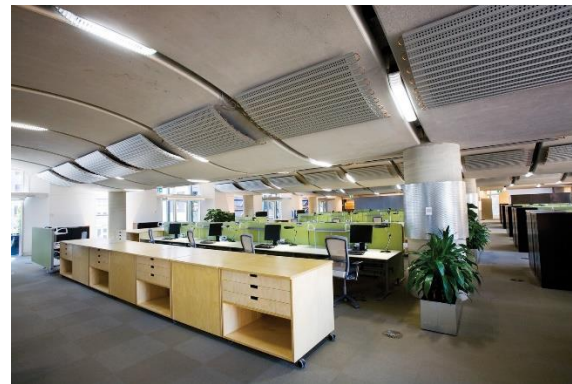
Fig [9]. The wavy ceiling that has the same function of soil in Termites mound.
